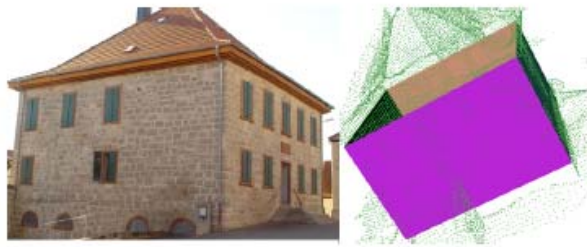
Figure 8: Left: Image of building consisting of four major walls standing on a slope. Right: The derived point cloud consists of 273 000 points, the four major walls were successfully detected, segmented and connected.
