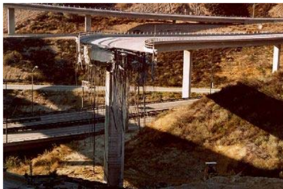
Figure 5-2: Highwaybridge in USA (Internet-Newsgroup)
