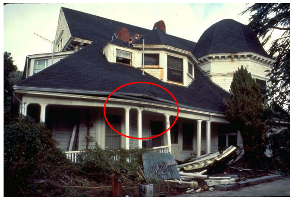
Figure 4-7: Loma Prieta, California earthquake in October 17, 1989 http://geohazards.cr.usgs.gov/eq/html/damage.html
