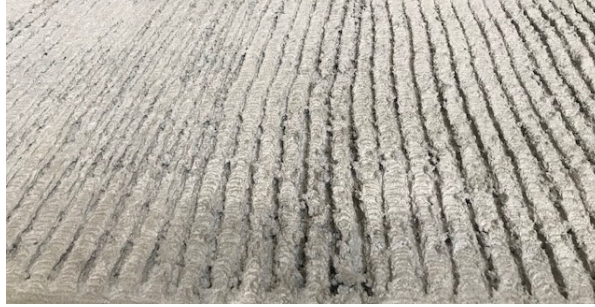
Figure 4.2.: roughened concrete surface before addition of fiber-reinforced layer
